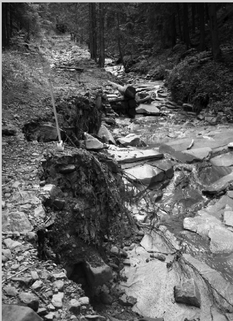
Fig. 9 Total destroyed section within the footpath in the Western Tatra Mts. An extreme rainfall ranging up to 104,2 mm on the 5 th of June 2007 resulted in temporary footpaths closing
